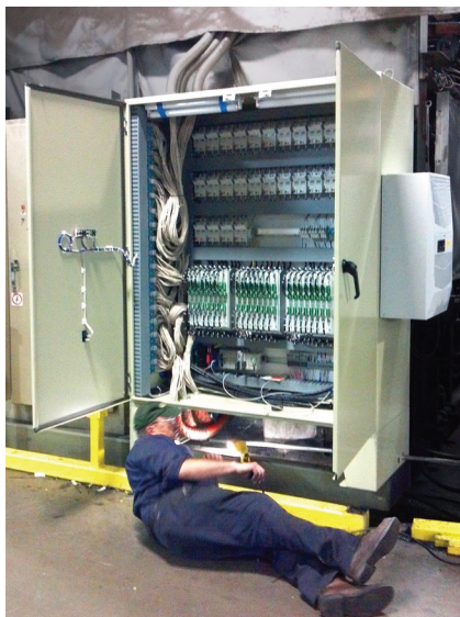
Control cabinet being installed by Weco on site
